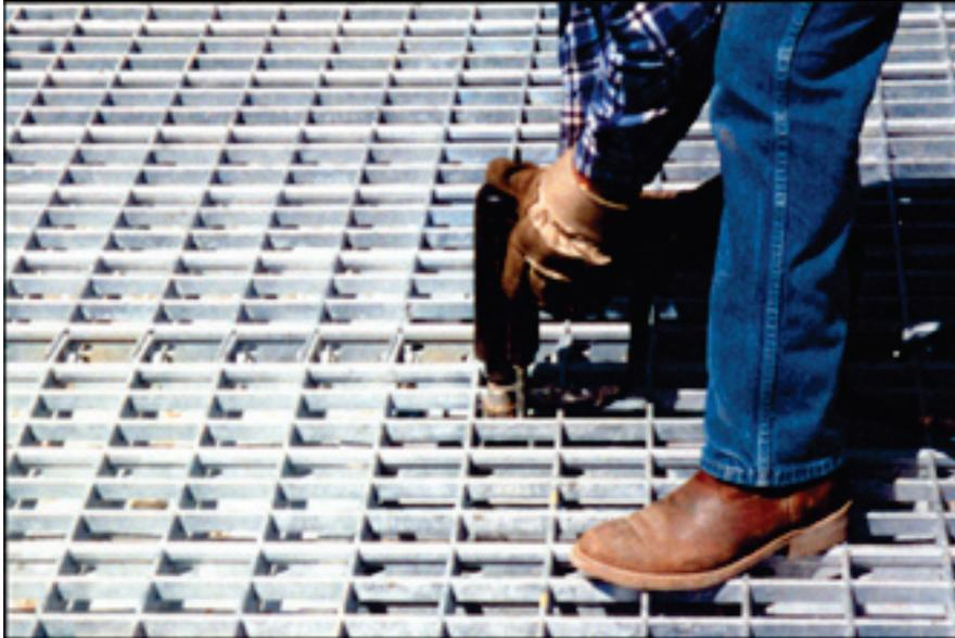
spacing must accommodate grid component spacing. Placing studs is accomplished through the use of automatic equipment, and can take place before or after grid panel erection.
