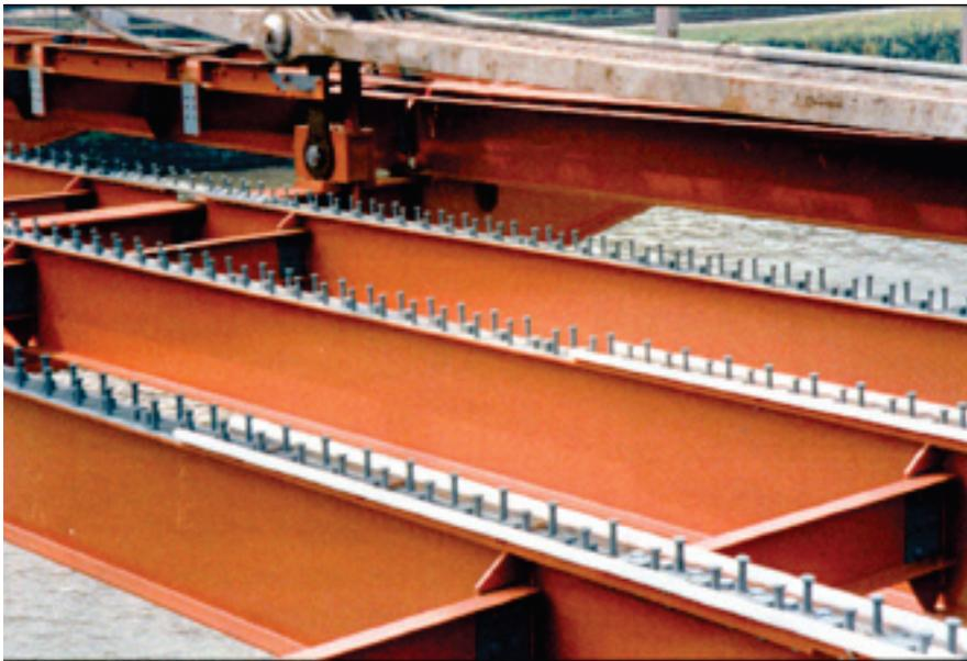
after they have been attached to the girders. In this situation, periodic weld equipment calibration and testing conducted on separate plates insures weld quality.
